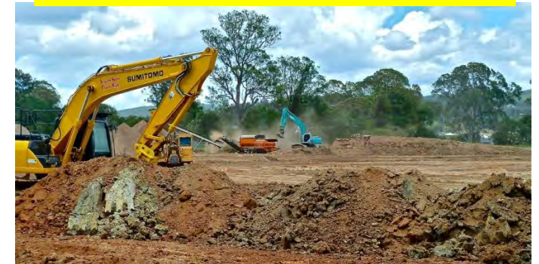
Construction on Farm Land
