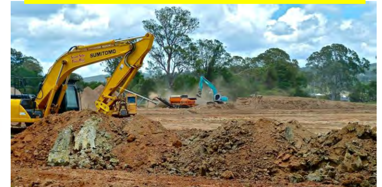
Construction on Farm Land
